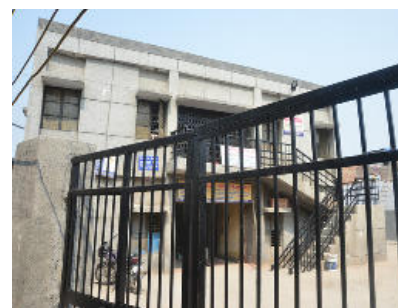
Social infrastructure in the area
